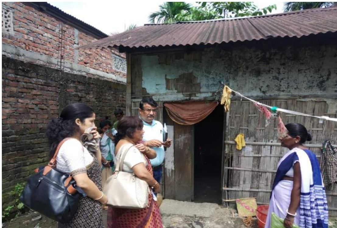
Fig. 1 Investigation by RRT team in affected house
